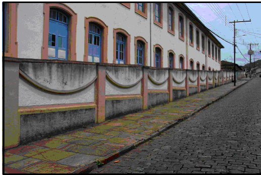
Figure 3. Curves on the wall of the school
